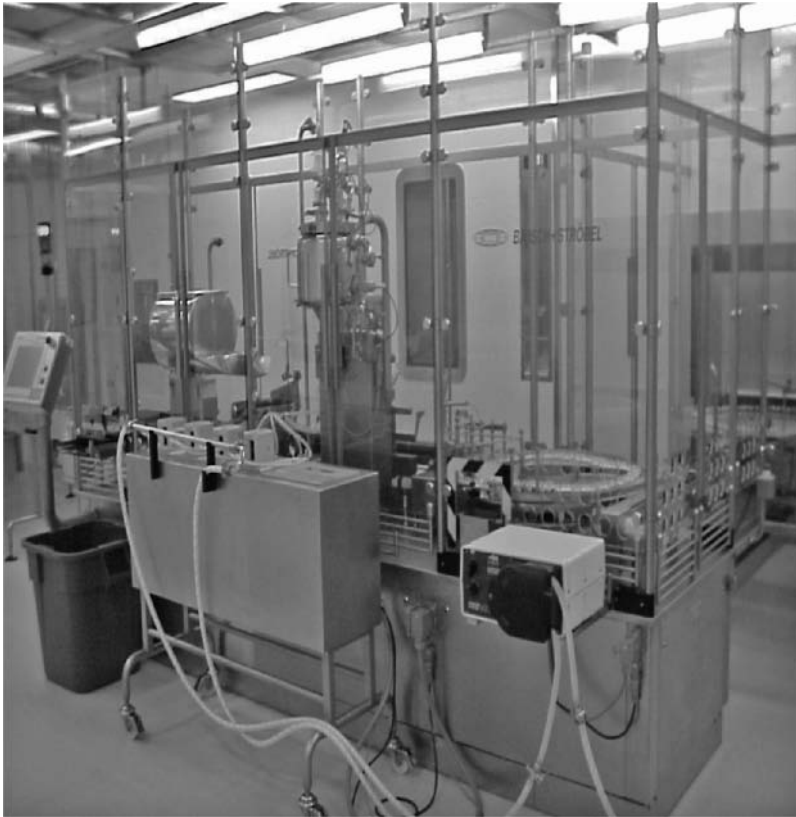
Figure 15-9 Filling line under vertical laminar airflow. Source: Courtesy of Baxter Healthcare Corporation.
