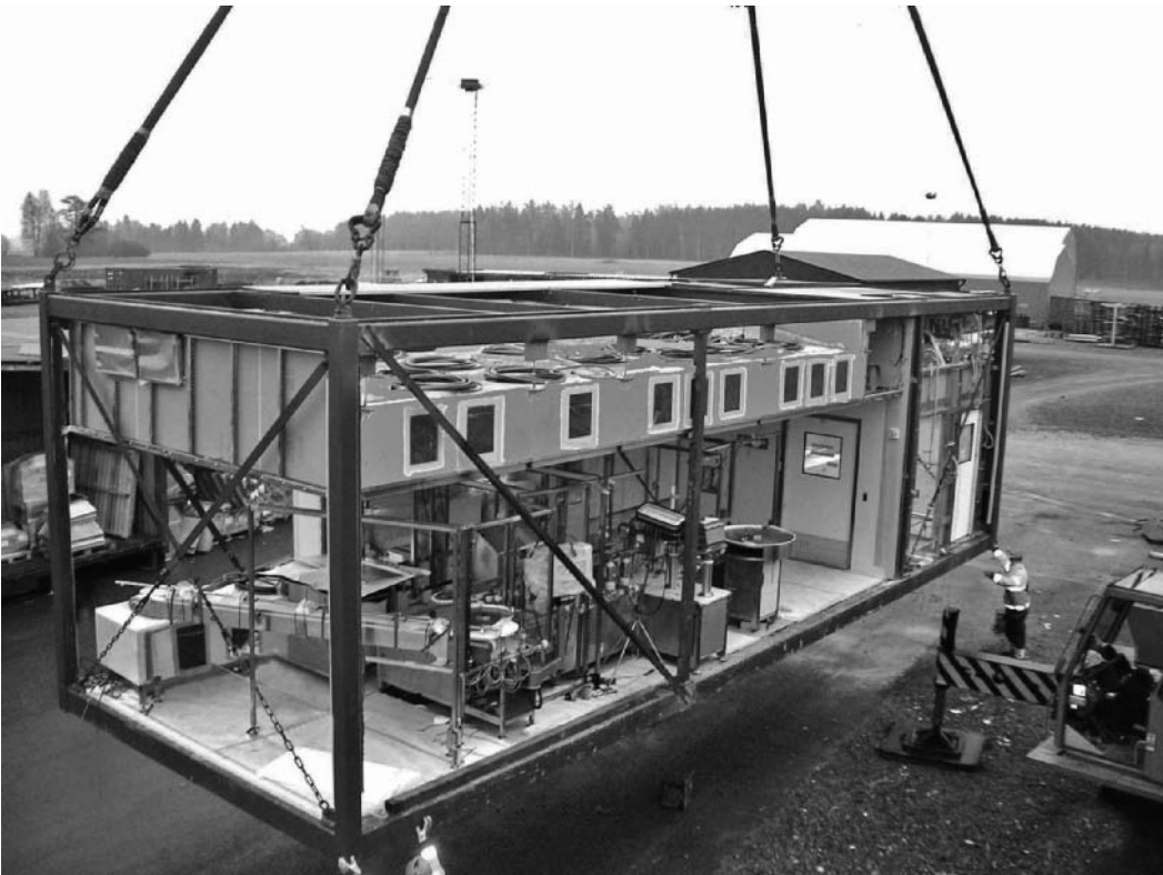
Figure 14-5 Example of a modular unit for a sterile manufacturing facility. Source: Courtesy of Pharmadule, Inc.
